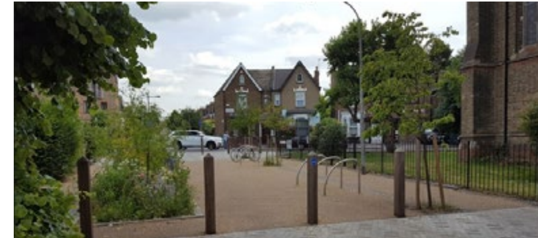
Northcote Road, Walthamstow – Modal filter with wooden bollards, planting, and cycle parking
