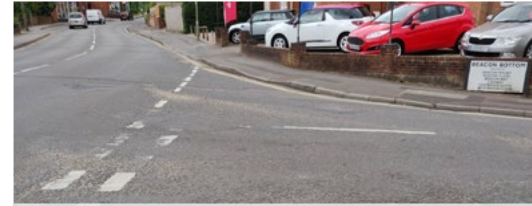
Z2.2.3 Beacon Bottom junction with Botley Rd
