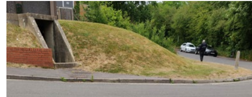
Z2.1.1 Swanwick Station accessibility issue
