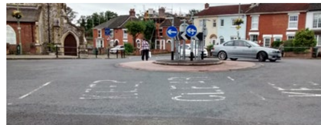
Z1.11.1b Hartlands Road roundabout clutter
