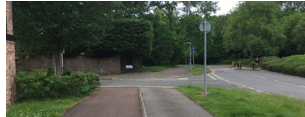
269.2.3b Existing shared facility along Centre Way
