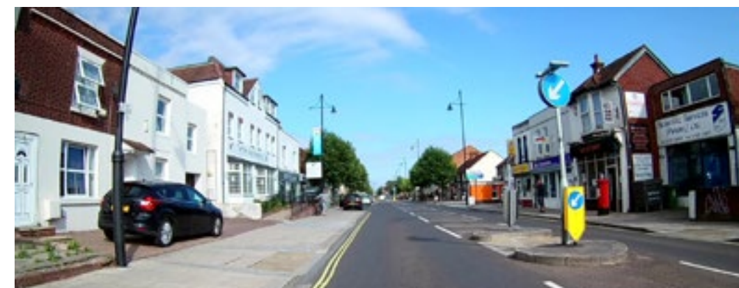
Z1.3.2 Crossing on West Street
