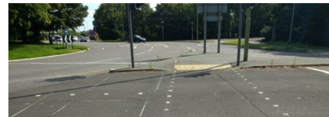
344.2.1 St Margarets Roundabout south western exit
