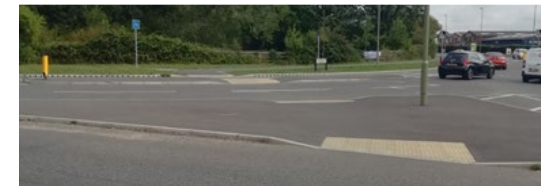
271.1.1 Longfield Avenue/Newgate Lane
