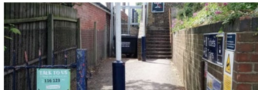
Z3.1.1 Stairs to southern platform of Portchester Railway Station
