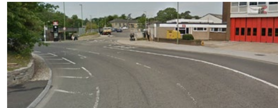
270.5.1 Station Roundabout north side
