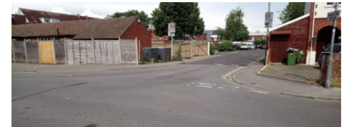
Z3.6.2 Southern Precinct car park access
