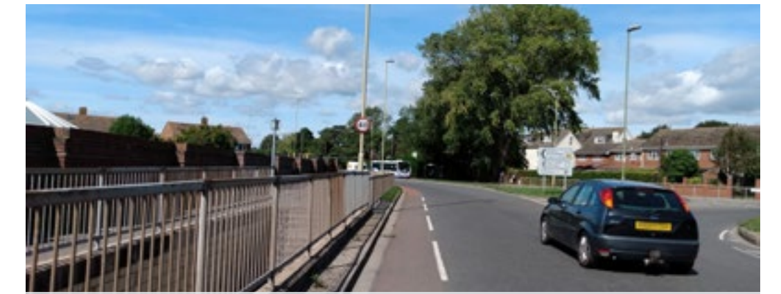
270.7.1 Cornaway Lane Roundabout
