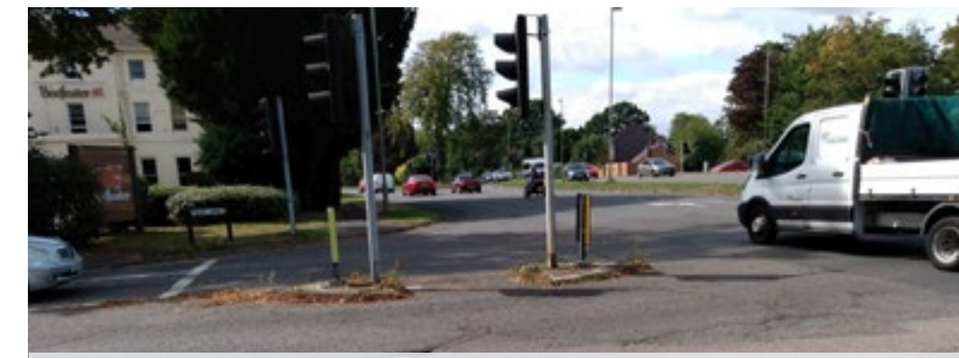
270.2.11 A27/Catisfield Road/Peak Lane signalised junction
