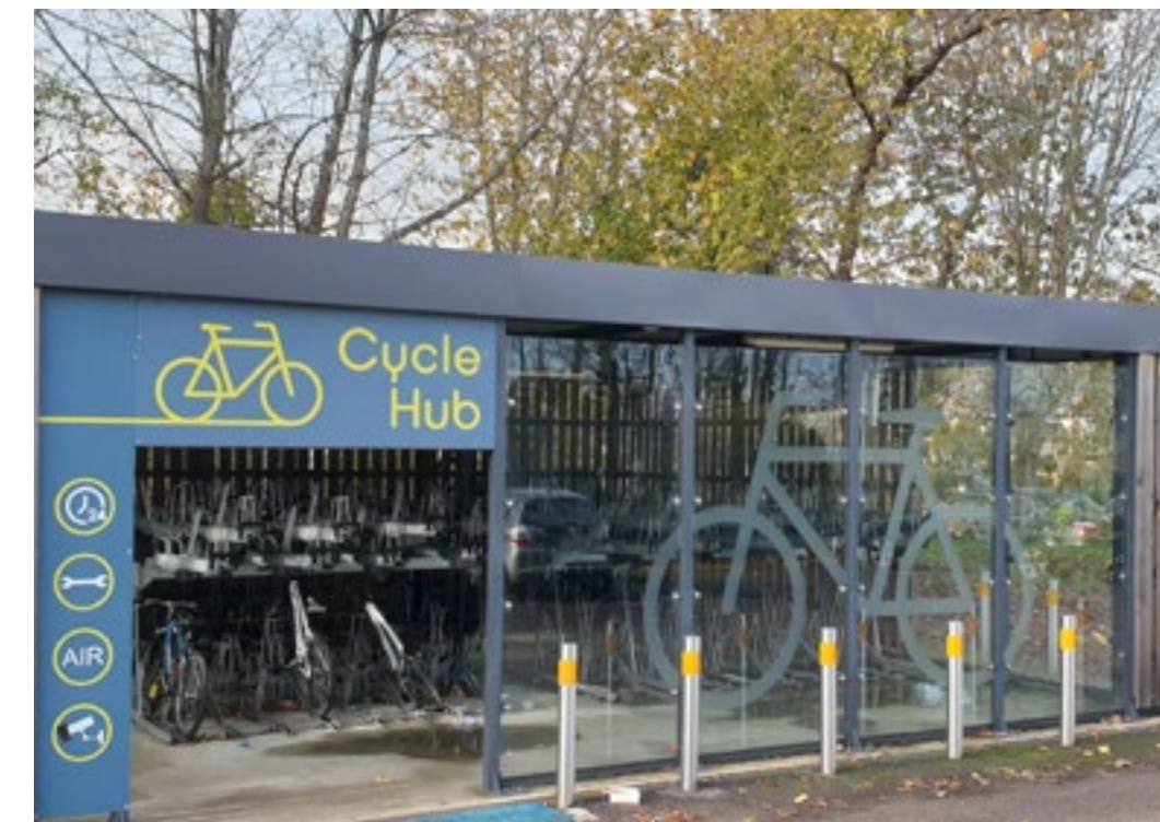
An example of cycle hub parking facilities – Winchester Train Station
