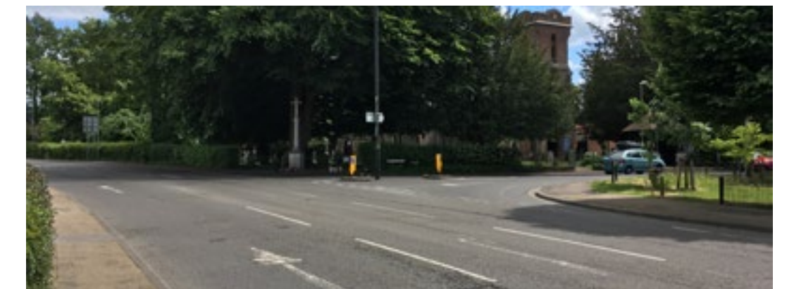
270.1.4 A27 Bridge Road – Barnes Lane junction
