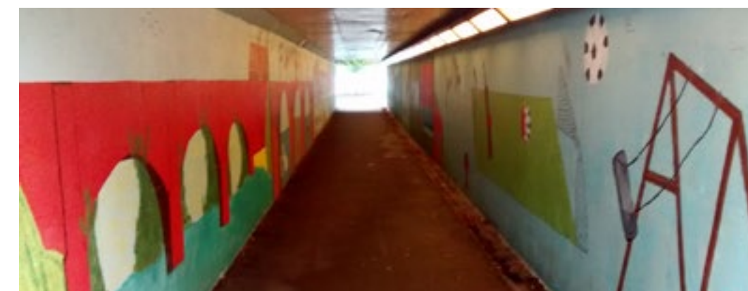
Z1.16.2b Bath Lane underpass
