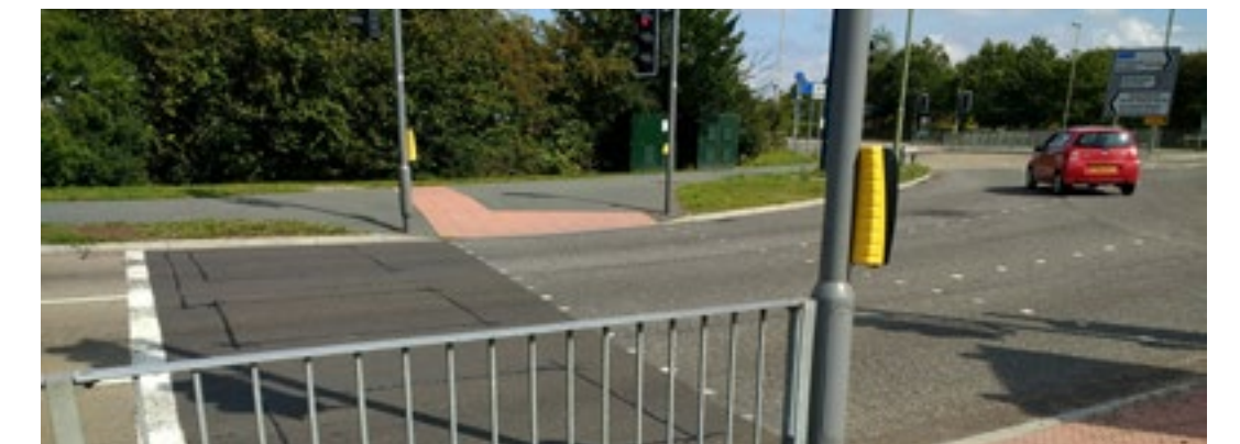
344.1.2 St Margarets Roundabout western entry
