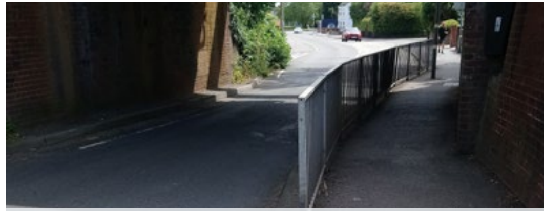
Z3.1.3 Route under railway bridge
