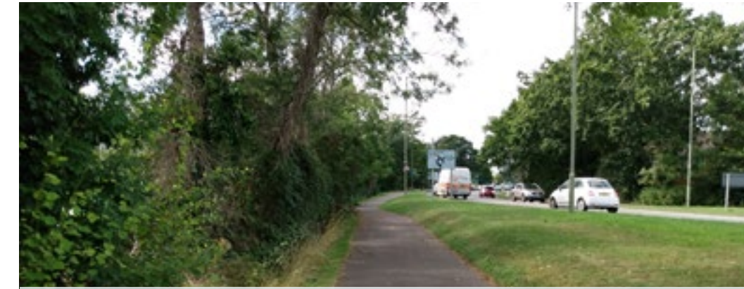
270.2.1 A27 Southampton Road shared path
