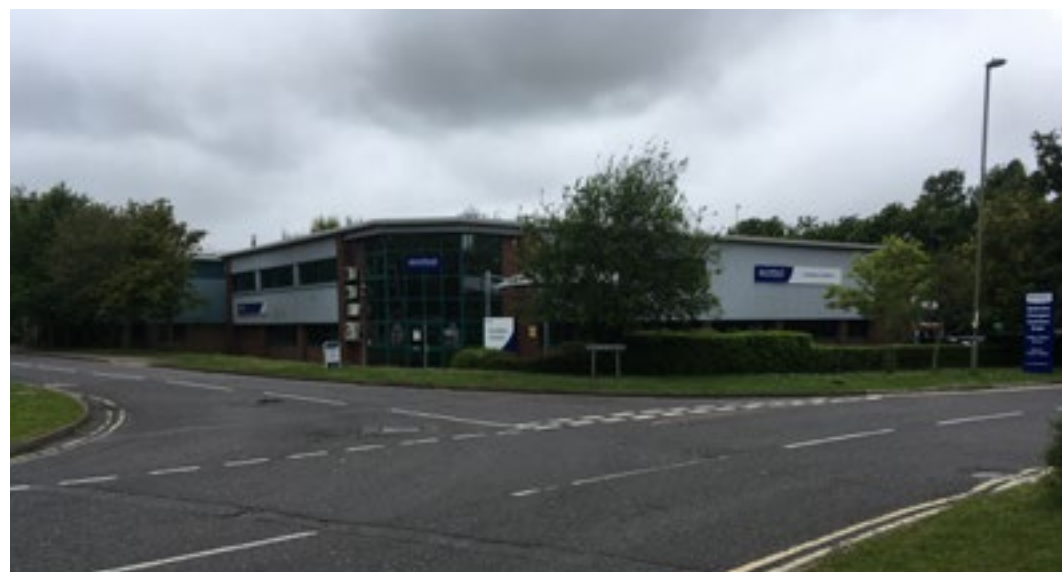
271.3.5 Little Park Farm Road/Whittle Avenue junction
