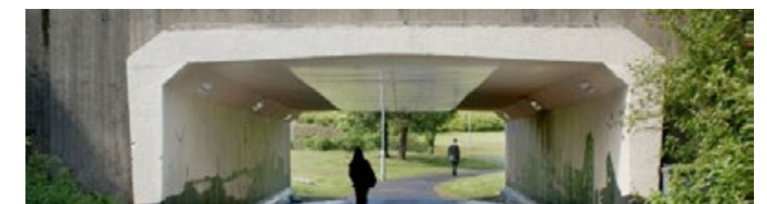
Well designed underpass by day/night
