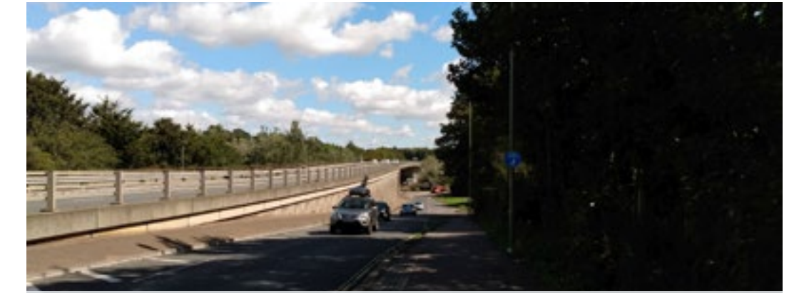
270.6.2 A27 Eastern Way On-slip
