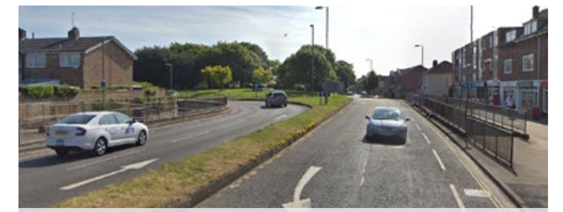
270.7.3 West Street Roundabout
