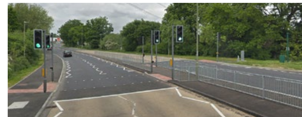
270.2.5 Crossing north of Titchfield Park Road
