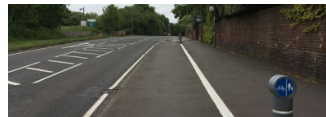
271.4.2 Shared footway running the eastern side of the A3051 Botley Road B
