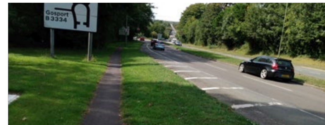
270.2.8 (b) Titchfield gyratory Westbound
